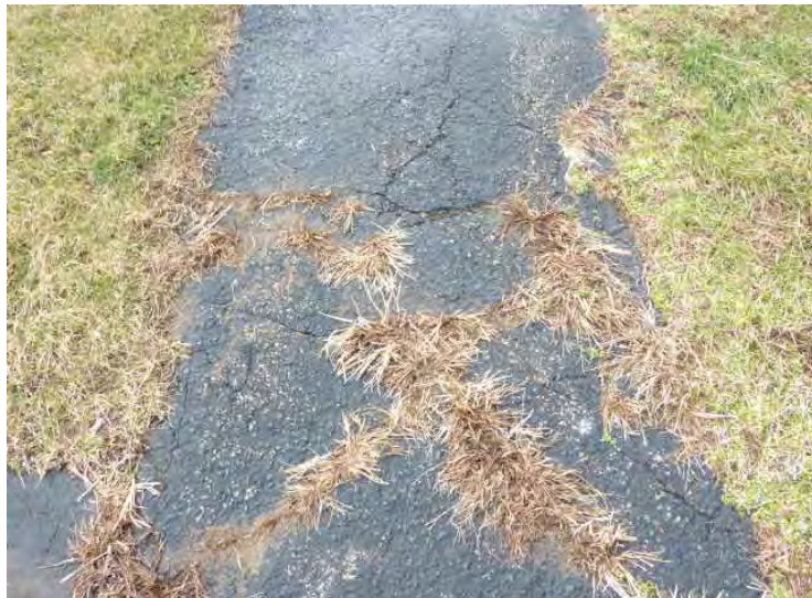
Typical asphalt walkway paving sub-base failure.
