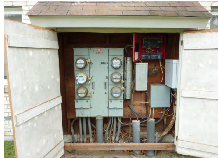
Typical electric/cable/fire alarm cabinets at each building are leaking and shown to be replaced.
