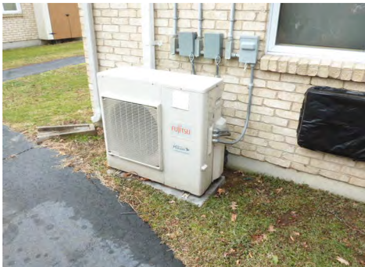
Typical split system unit heat pumps only at the 2 accessible units.
