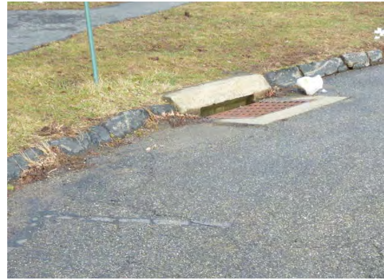
Damaged curb to be replaced when the asphalt overlay takes place early in the plan.
